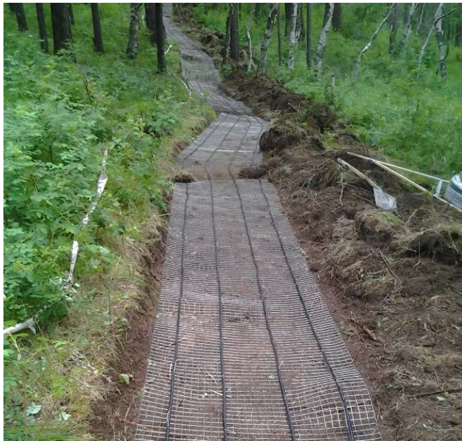
Figure 1. Underground Sensor Cable Installation
